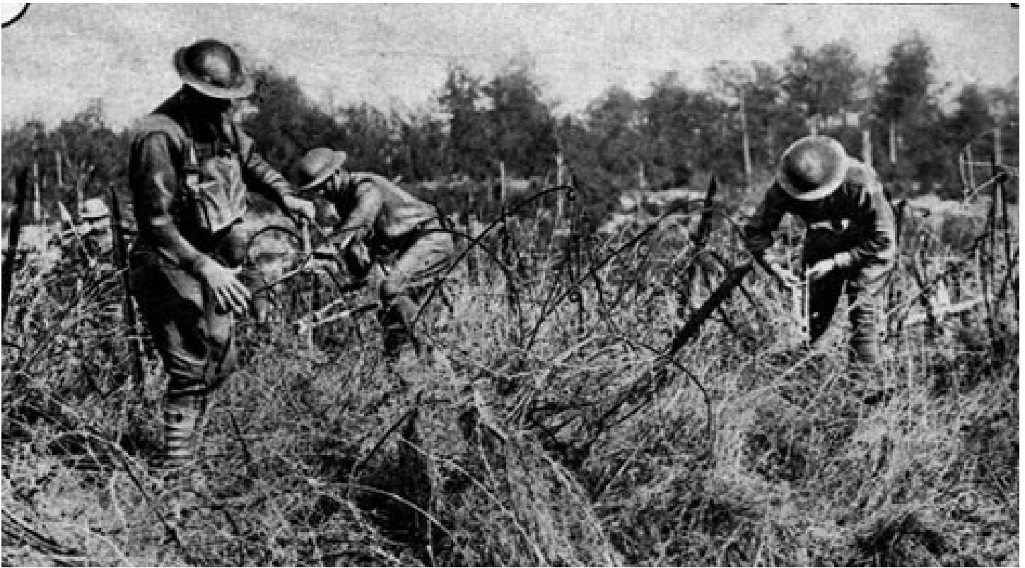
107th Engineers Cutting wire
